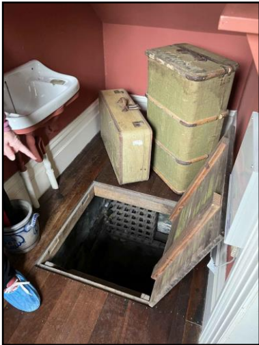
Former Scullery converted to wine cellar.
