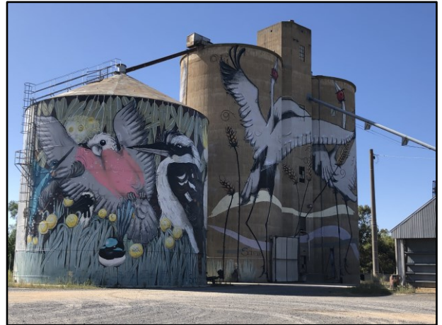
Tungamah Silos, Wow the detail was impressive.
