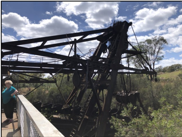
The buckets & booms were operated by 14 electric motors consuming massive 670Kw of power.
