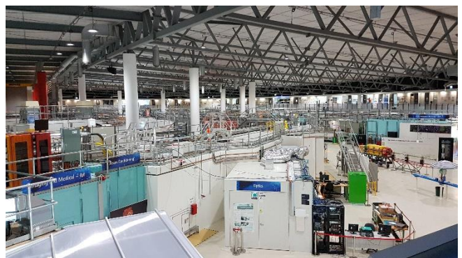
Overview of Synchrotron facility.
