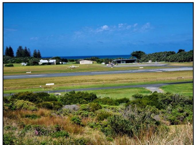
View of Airport from Transit hill track.
