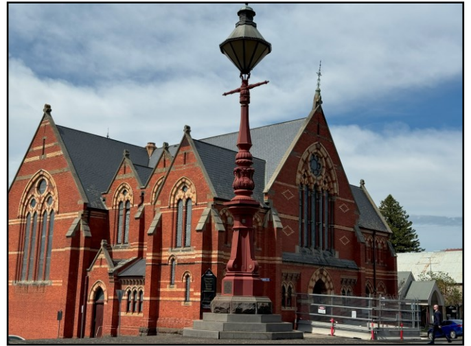
Ballarat Uniting Church with original Gas lamp.
