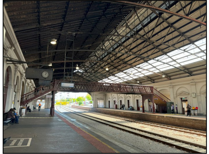
Railway platform showing the pedestrian overpass.
